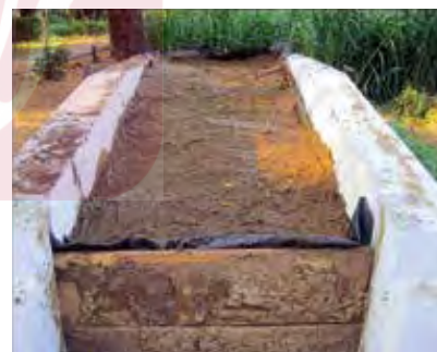
Fully sealed silo pit
